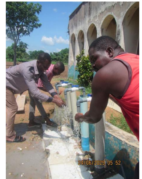
The water is flowing for the first time at Ishiokoma Health Center
