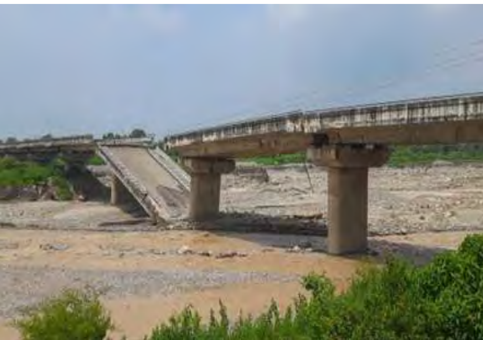
This bridge over the Malan River collapsed on 13 July 2023 during flooding of the river
